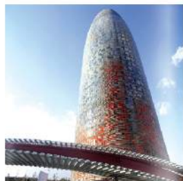
Torre Agbar, Barcelona, Spain
